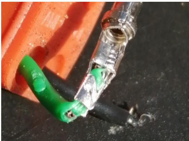
Loadcell wire cut inside connector, at the terminal crimp
